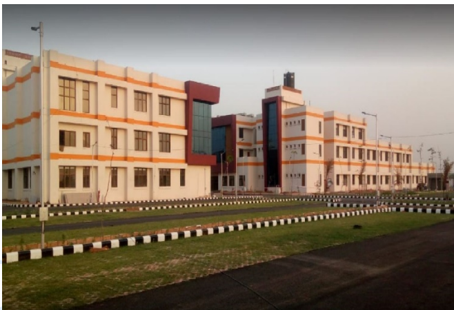
Newly constructed, MSME – TC Bhiwadi
